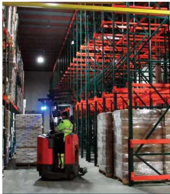
Rack demolition crews kept just one sector ahead of the installation crews, keeping the number of out-of-commission storage bays to a minimum.
